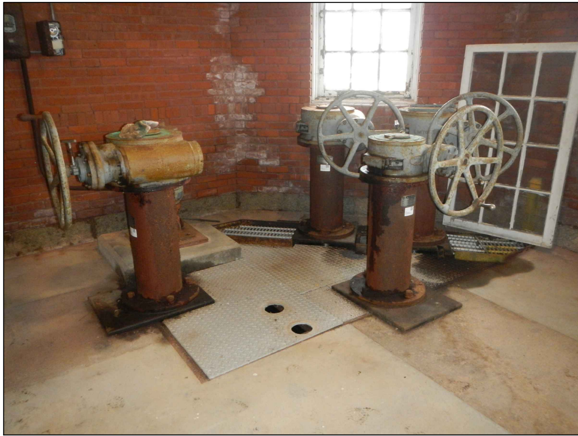
PHOTO 7 OUTLET STRUCTURE (INTERIOR - EXISTING VALVE OPERATORS ON NORTH SIDE)
