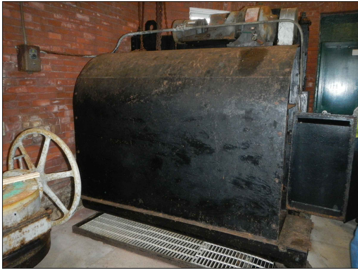
PHOTO 6 OUTLET STRUCTURE (INTERIOR - EXISTING MECHANICAL SCREEN)
