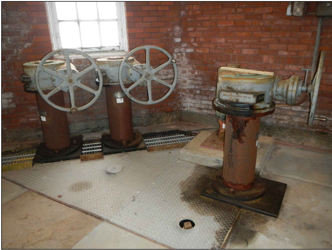
PHOTO 8 OUTLET STRUCTURE (INTERIOR - EXISTING VALVE OPERATORS ON SOUTH SIDE)
