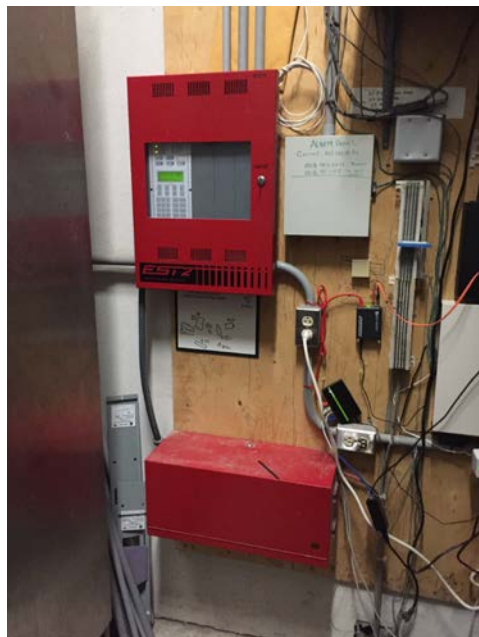
Aquatics Facility EST2 FACP and battery box below.
