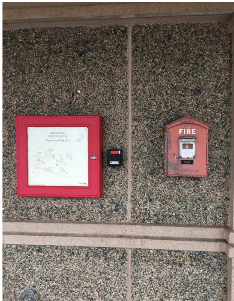
Administration Building Remote Annunciator, Master Box and Key Box
