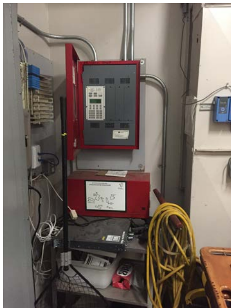
Animal Care Facility EST2 FACP and battery box below
