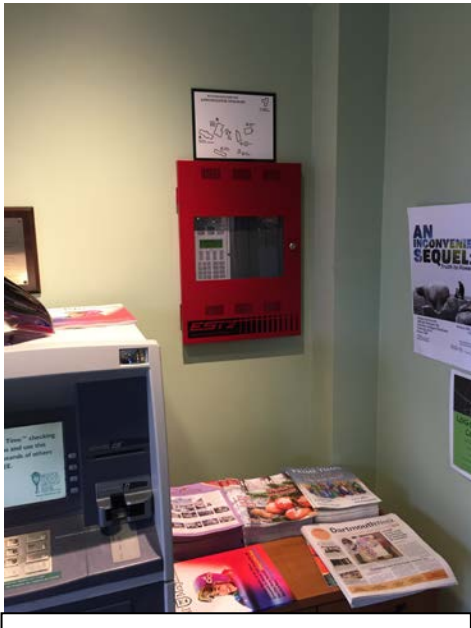
Administration Building EST2 FACP. Battery box in adjacent room behind FACP.
