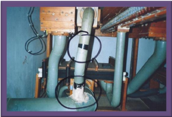
Emergency air leaks repaired with electrical tape and putty.
