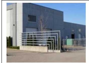
Screening of service and loading areas
