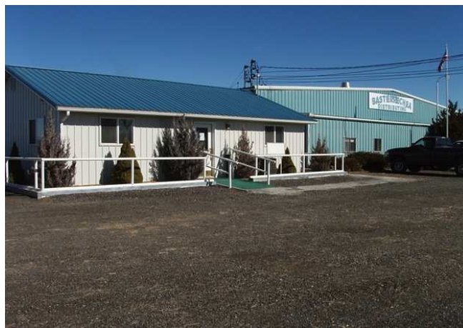
Figure 2 - Existing Facility in Gooding, Idaho
