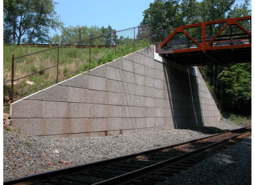
LIRR Double Track Project Ronkonkoma to Farmingdale Retaining Wall Finishes Figure 2-14
