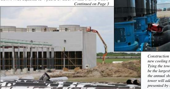
Construction is nearing completion on the new cooling tower at Golden Grain Energy. Tying the tower into the rest of the plant will be the largest project undertaken during the annual shutdown June 20-24. The new tower will address quality and safety issues presented by steam with the previous cooling tower, in addition to meeting plant capacity.
