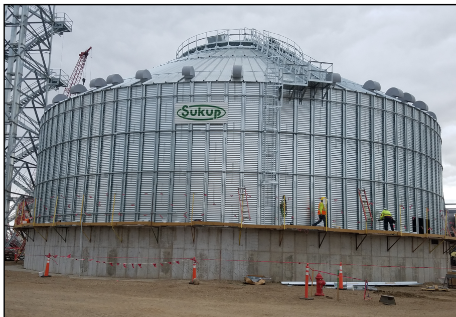
Sukup Manufacturing crews have a good start on this 750,000 bushel grain storage bin on the Ringneck Energy site.
