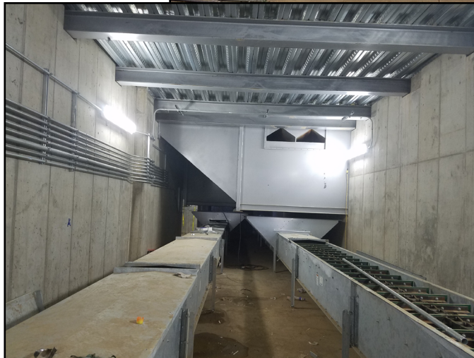
Above: The process building is taking shape. Left: The hopper and conveyor are in place in the grain receiving area.
