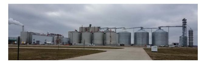
We plan to maintain our quest towards higher production rates in FY 2017 by continuing to invest in the plant. The Board has approved projects to add another fermenter, add an additional cooling tower cell and a beer-degasser to the process. These projects are expected to assist in increasing production rates and are expected to be complete by the end of FY 2017. The projects are expected to cost approximately \$4,356,000.
