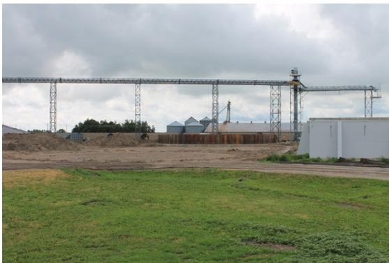
The project at Orleans is moving forward at a pace which is a little slow due to excess rain. The pilings are complete for all three bins with the pile cap being complete on bin #1. The outer walls on the above ground tunnel on bin 1 should be complete by Friday (6-29-18) with backfilling to start the following Monday. The expectation would be to have the first one backfilled by the end of the week to be ready for the cap and soon after that to start on bin #2 to repeat the process.
