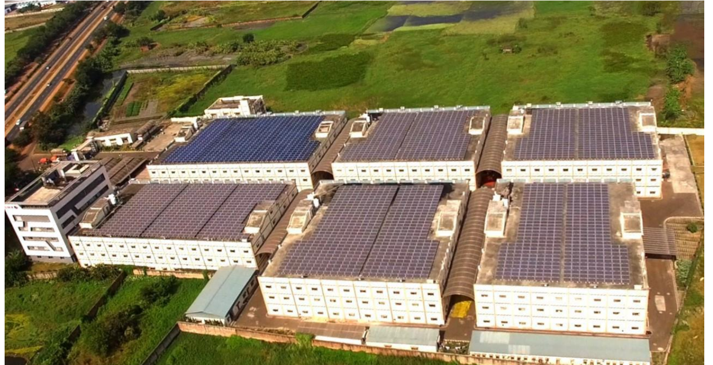
Rooftop solar power plant at Dankuni unit
