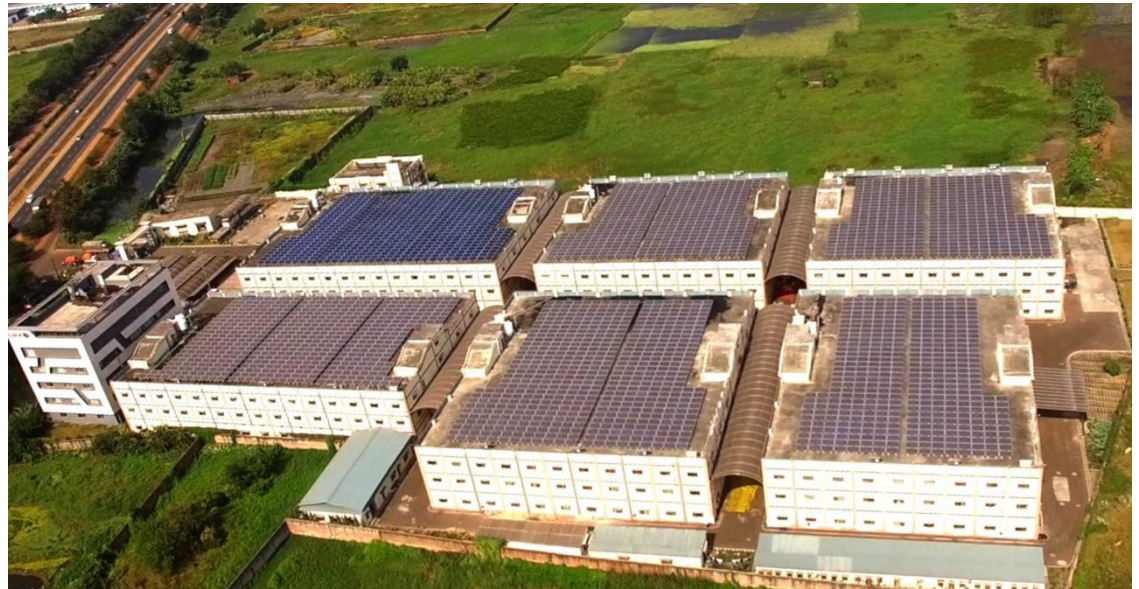
Rooftop solar power plant at Dankuni unit
