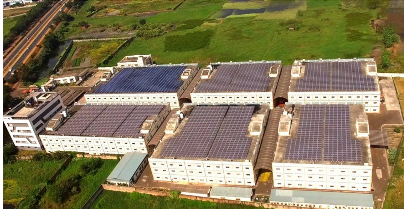
Rooftop solar power plant at Dankuni unit
