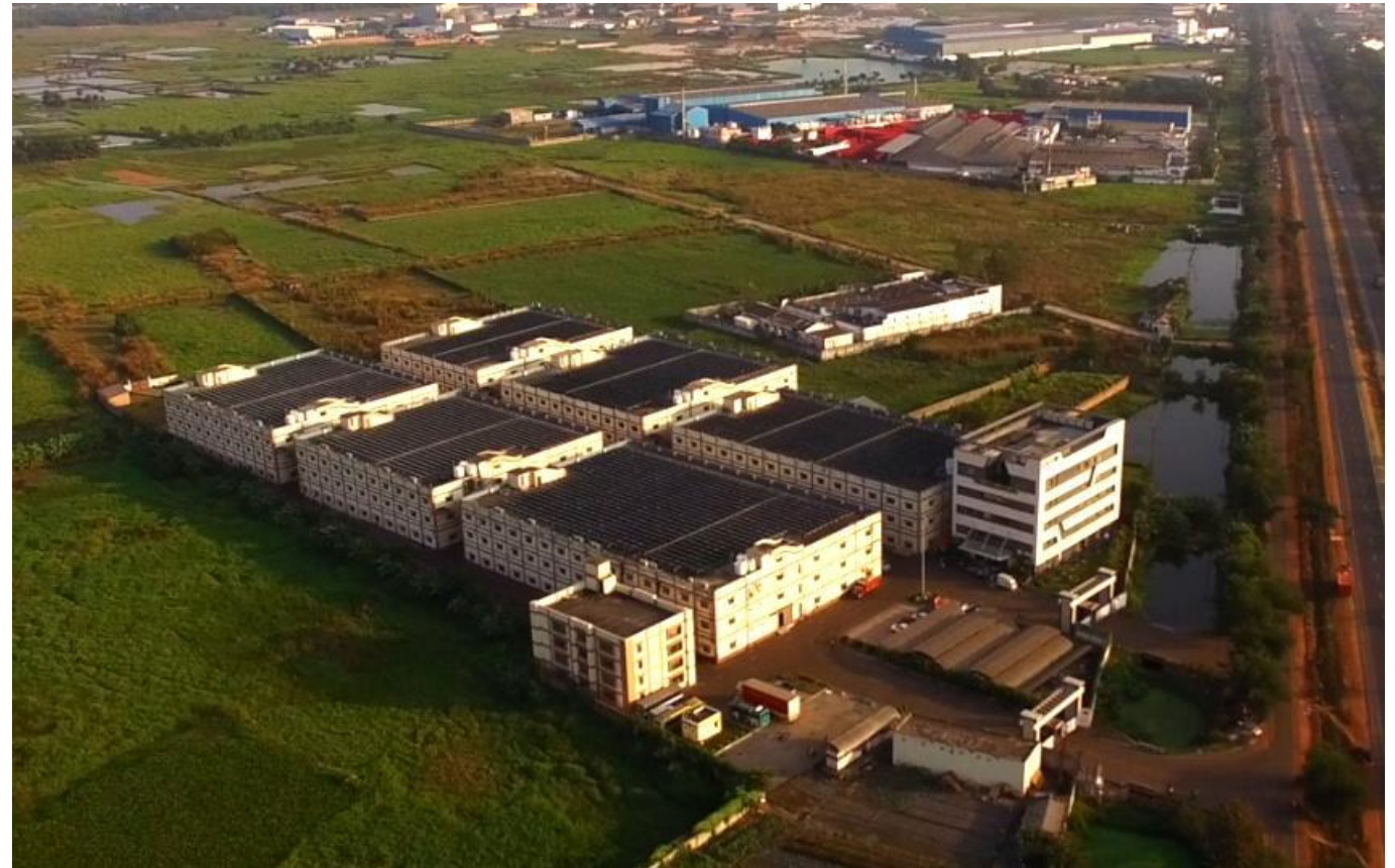
Rooftop solar power plant at Dankuni unit
