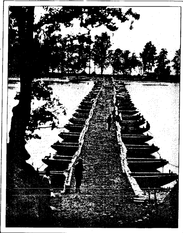
PONTOON BRIDGE AT DEEP BOTTOM, VA.
