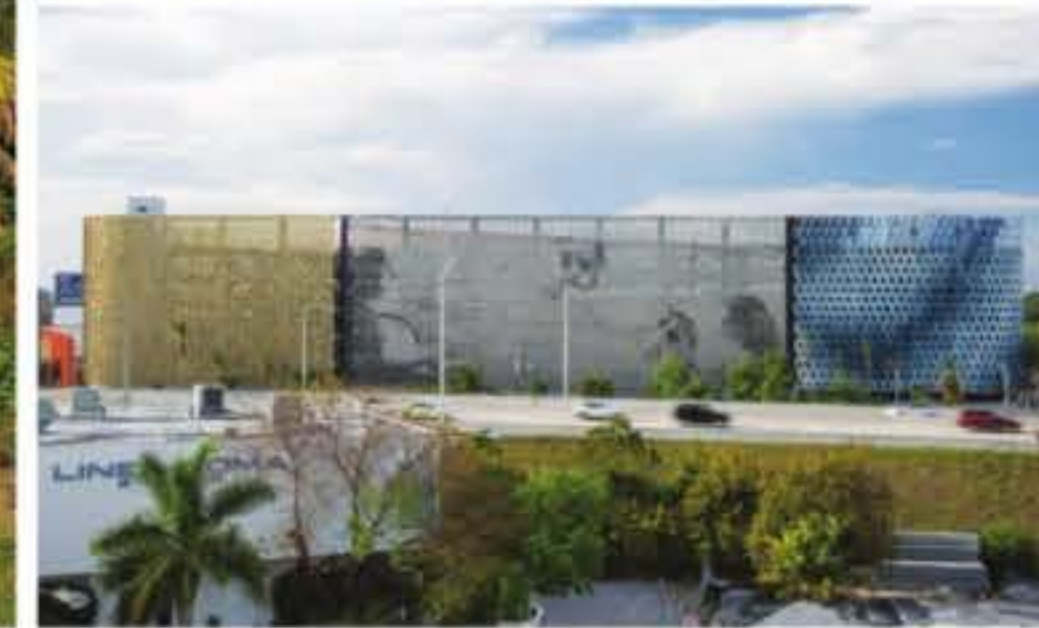
MIAMI DESIGN DISTRICT CITY GARAGE, 2015 ← ↑ Folded fin cut-outs in panels of gold titanium-coated steel create an attractive aesthetic on the exterior while diffusing the sunlight that streams in. ← The unique project merges three distinct facades, with Leong Leong's contribution on one end and San Francisco firm IwamotoScott's on the other. The work of artist John Baldessari adorns the centre panel.
