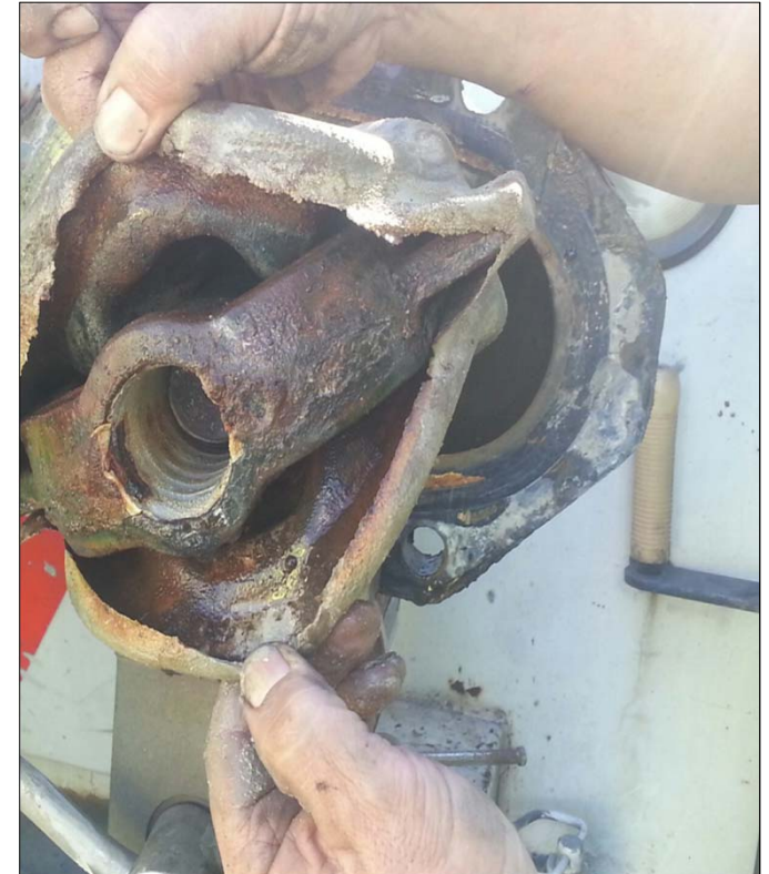
Old Valve that was Repaired
