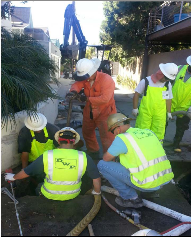
Removal of Water Valves
