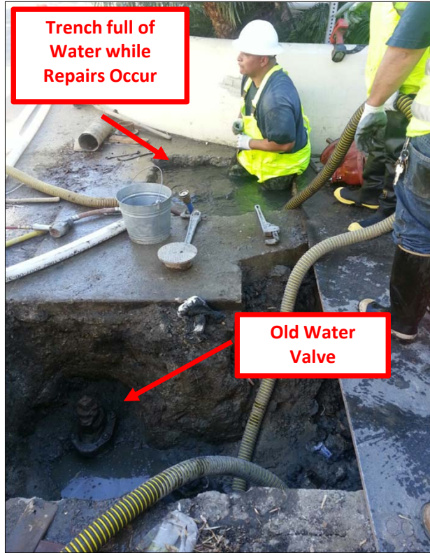
Repair of Water Valves
