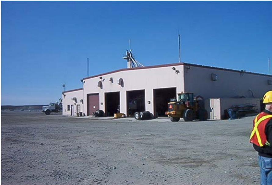
Garage (front) and process building (rear).
