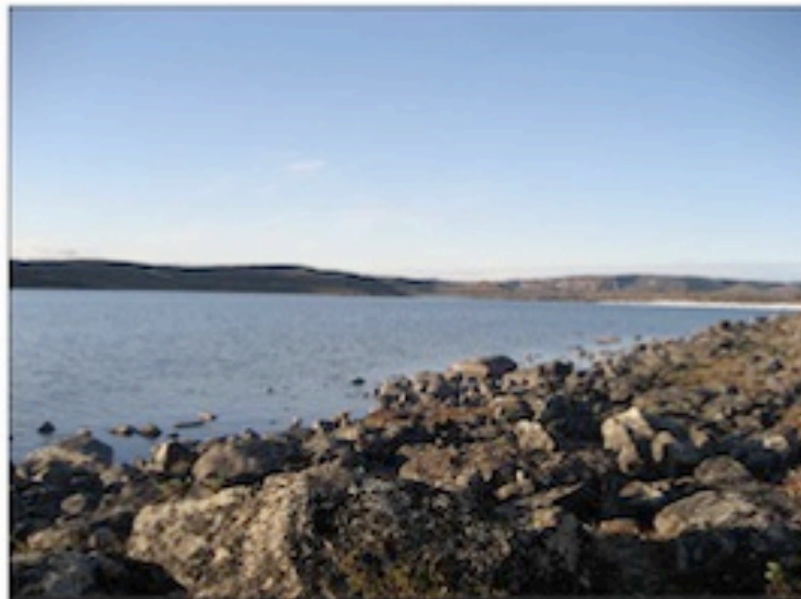
PHOTO 58 – Looking upstream from gauging station BR137 on Aug 2, 2008. (Discharge = 10 m 3 /s)
