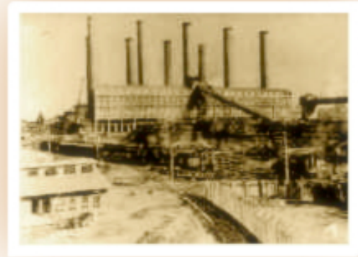
DuPont Powder Plant c. 1917 Old Hickory, TN
