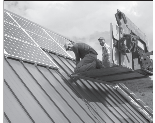
Luke (left) and John Kahle install photovoltaic panels.
