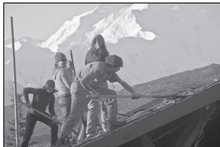
Staff ripping shingles from Potlatch.
