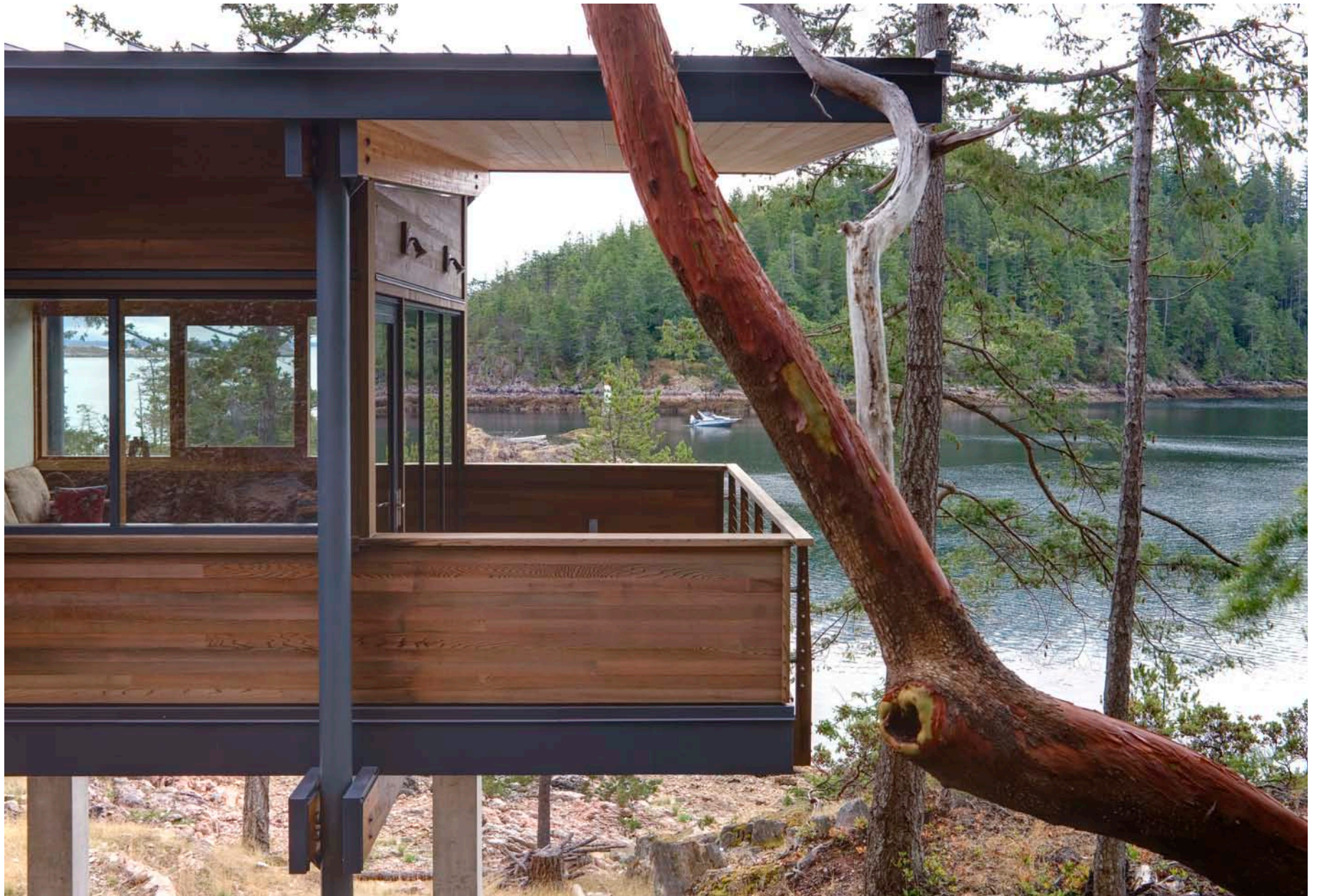
cantilevered deck off study
