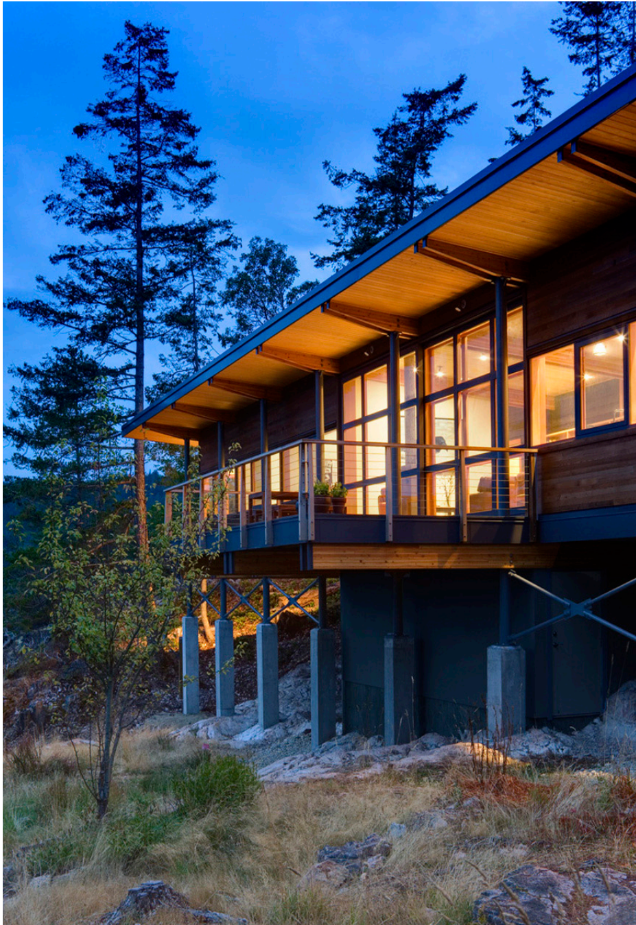
large deck cantilevered from great room
