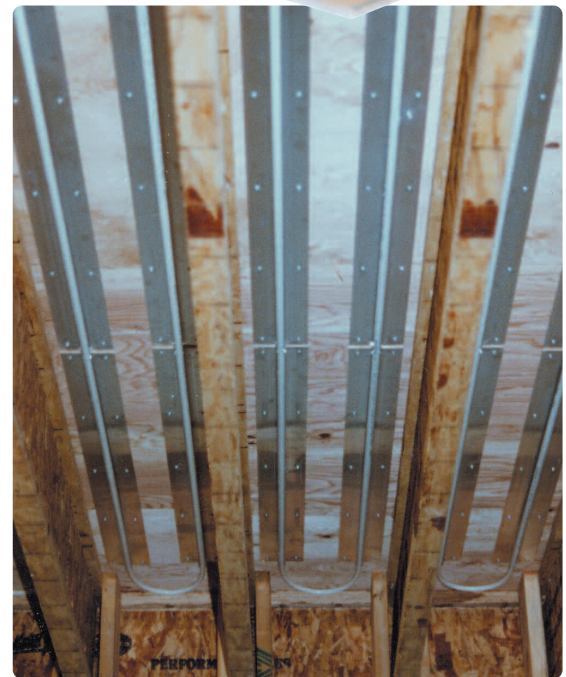
Wirsbo hePEX plus tubing easily and securely snaps into the Joist Trak channel for faster installations without extra fasteners.
