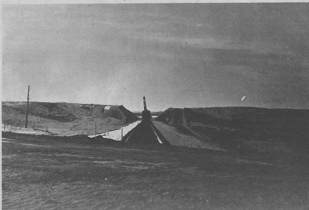
New railroad spurs have already been built into Decker, Montana, (shown here) and to a strip mine south of Gillette, Wyoming. New spurs proposed or under construction will go to Sarpy Creek in Montana and link Douglas and Gillette, Wyoming, through the Powder River Basin.
