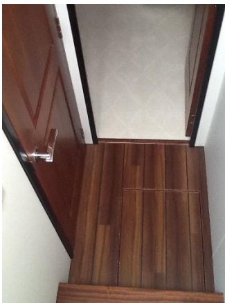
Custom lower level flooring and carpet
