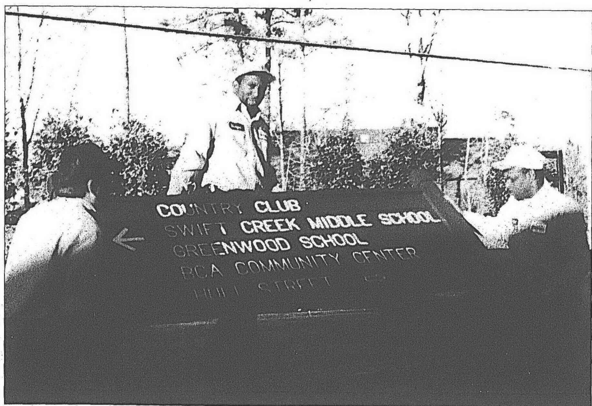
Photo by Wendy Parker Maintenance employees, from left, Charles Cashion, Dwayne Patterson and Garland Bannister work together in repairing many of Brandermill's signs.
