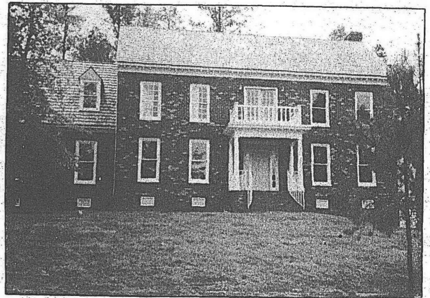
This Tomac home is nearly ready for the opening date of Homearama. Workers are still busy landscaping and putting the finishing touches on the interior.
