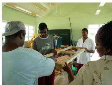
4. Assemble frame with wood glue and screws
