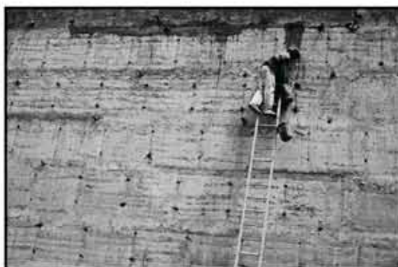
Rebuilding the Wall Around Taroudant, 2011
