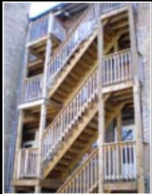
Main Rear Porch Rebuilt in 2002
