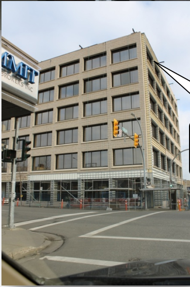
Scotia Bank building is being refaced with stone.
