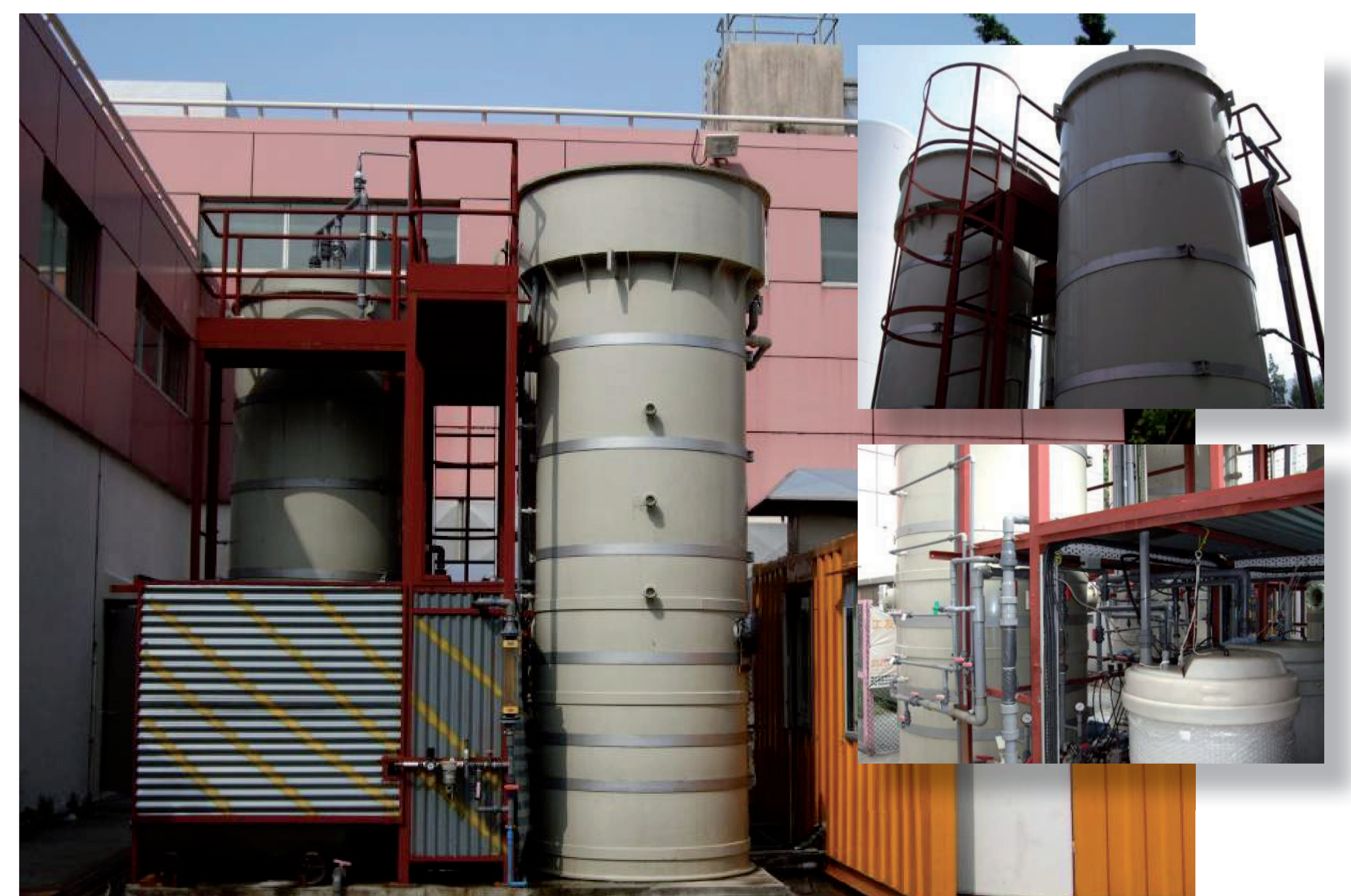
Figure 3. A pilot plant, operating successfully, using the SANI process in Hong Kong to treat municipal wastewater containing significant amounts of seawater [Lu et al. 2010].
