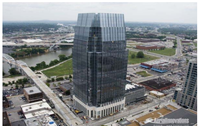
The Pinnacle at Symphony Place, 29-story Class A office tower
