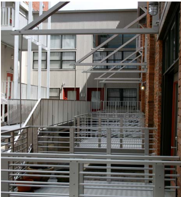
Interior Courtyard at Art Avenue Lofts - 5th Avenue
