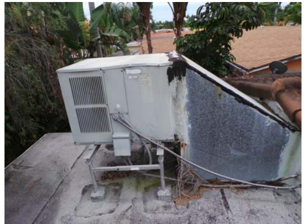
Replace AC system
