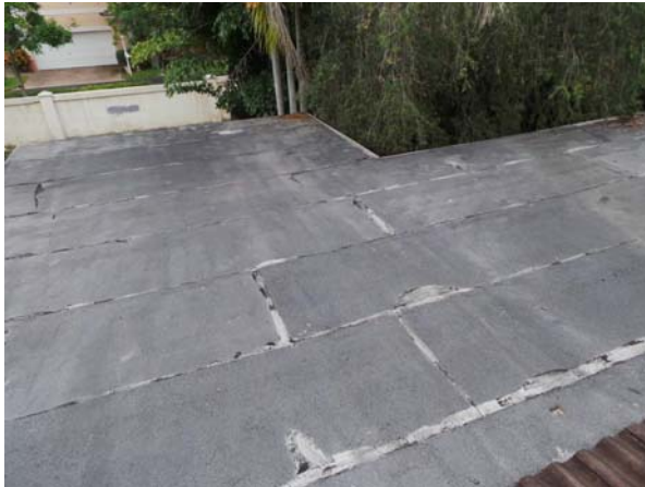
Replace flat roof
