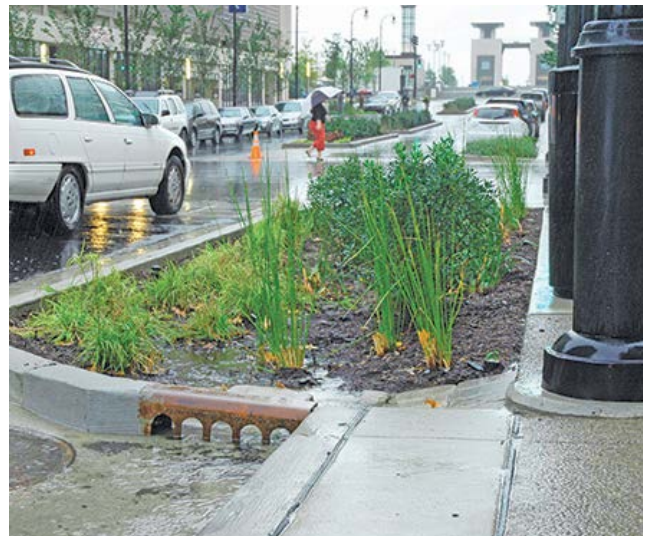
BULB-OUT PLANTER WITH STORMWATER INLET
