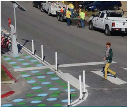
PAINTED CURB EXTENSION
