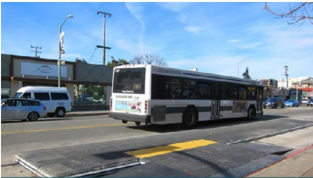
TEMPORARY TRANSIT ISLAND WITH BIKE LANE
