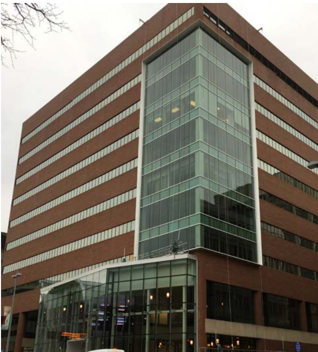
FACADE RETROFIT PARTIALLY TRANSFORMS SCALELESS BUILDING WITH A 3-PART BUILDING COMPOSITION AND A STOREFRONT WITH MAXIMIZED CLEAR GLASS
