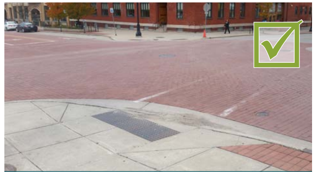
PAVER BANDING AT ACCESSIBLE CURB RAMP
