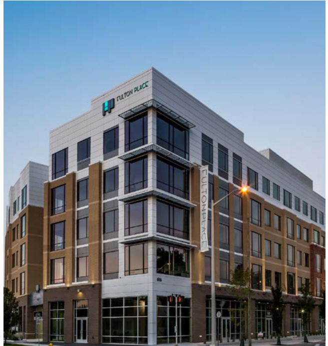
NEW CONSTRUCTION THAT HAS A VERTICAL PATTERN, 3-PART COMPOSITION, SIMPLIFIED MATERIAL PALETTE, HORIZONTAL EXPRESSION LINE AT STOREFRONT, AND A VERTICAL WINDOW PATTERN
