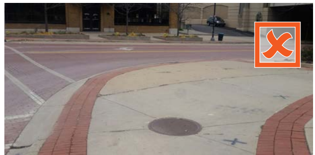
PAVER BANDING EXTENDING THROUGH ACCESSIBLE CURB RAMP
