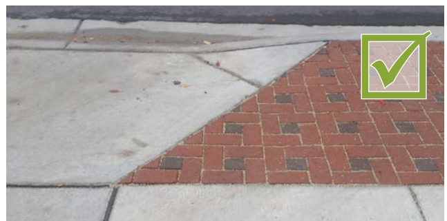
PAVER BANDING TERMINATING INTO DRIVE ENTRANCE FLARE
