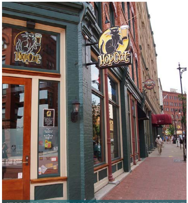
STOREFRONT THAT INCLUDES THE FIVE STOREFRONT DESIGN ELEMENTS (BULKHEAD, DISPLAY WINDOW, ENTRANCE, TRANSOM, & BEAM) + HUMAN SCALED MATERIALS AND DETAILS + ADDED COLOR ACCENTS
