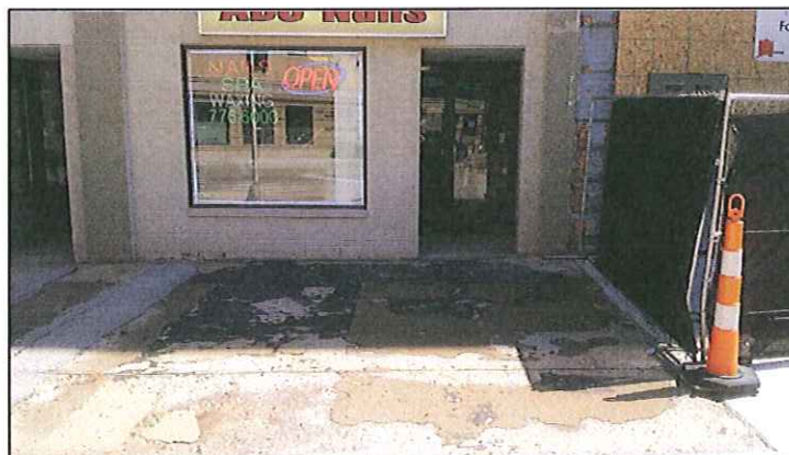
Figure 1: Picture of existing Areaway Cap
