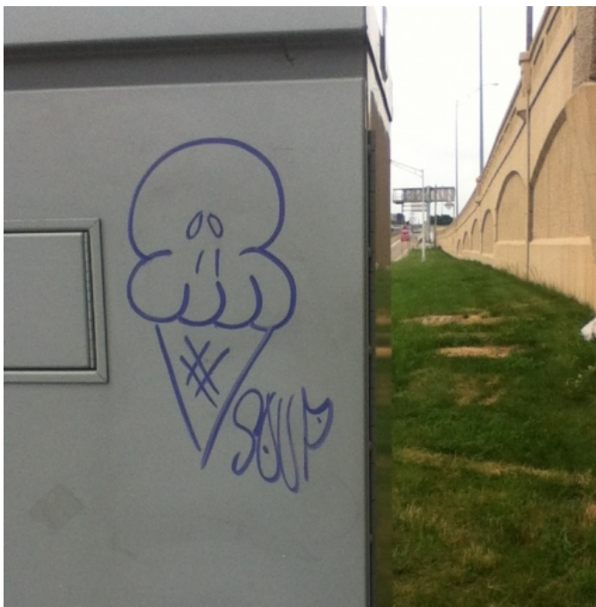
Utility Box Before...
