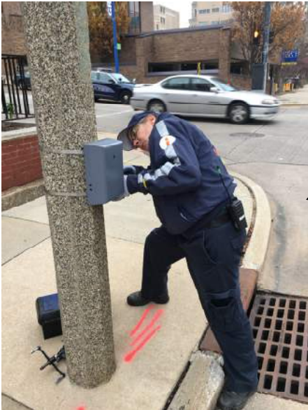
Ellen installs a pedestrian counter on Lyon & Division.
