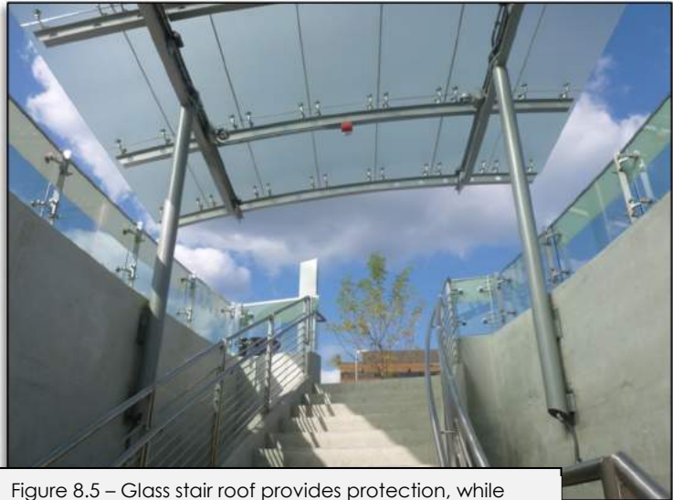
Figure 8.5 – Glass stair roof provides protection, while allowing natural light to reach lower parking levels.
