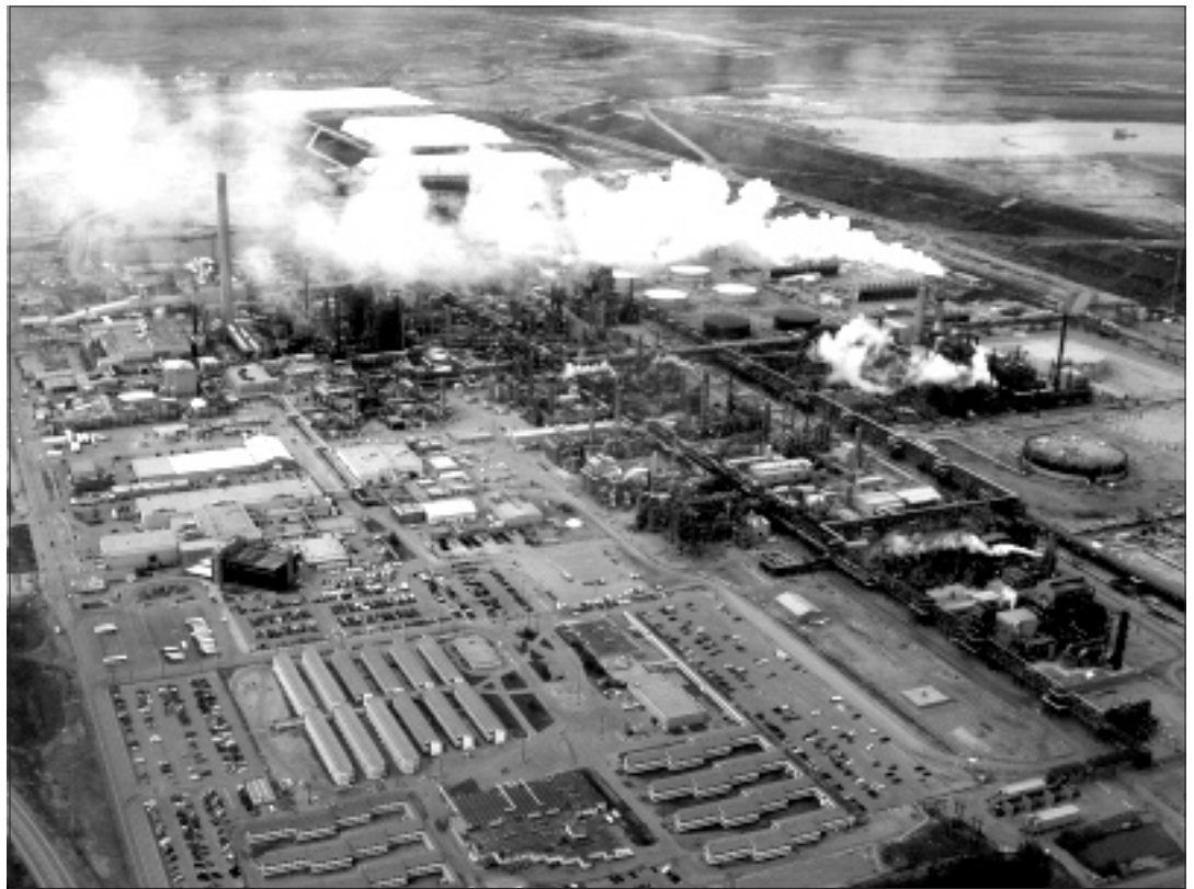
Tar sands production is set to increase as conventional oil reserves are depleted.
