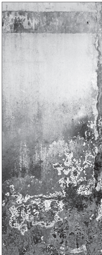
Sub-standard construction means that in addition to crowded conditions, mildew is a major problem in on-reserve housing. oy gen CC2.0
