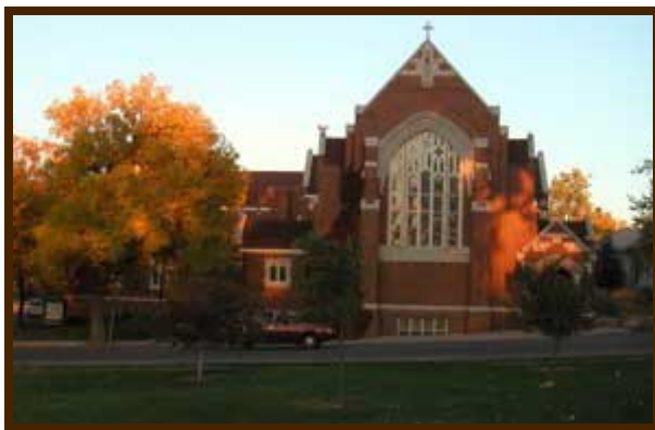
For nearly 90 years, St. Mark's beautiful brick church has been loved by members and the community. Generous bequests, a plate & pledge set-aside and a very dedicated building committee have kept the structure in excellent shape.
