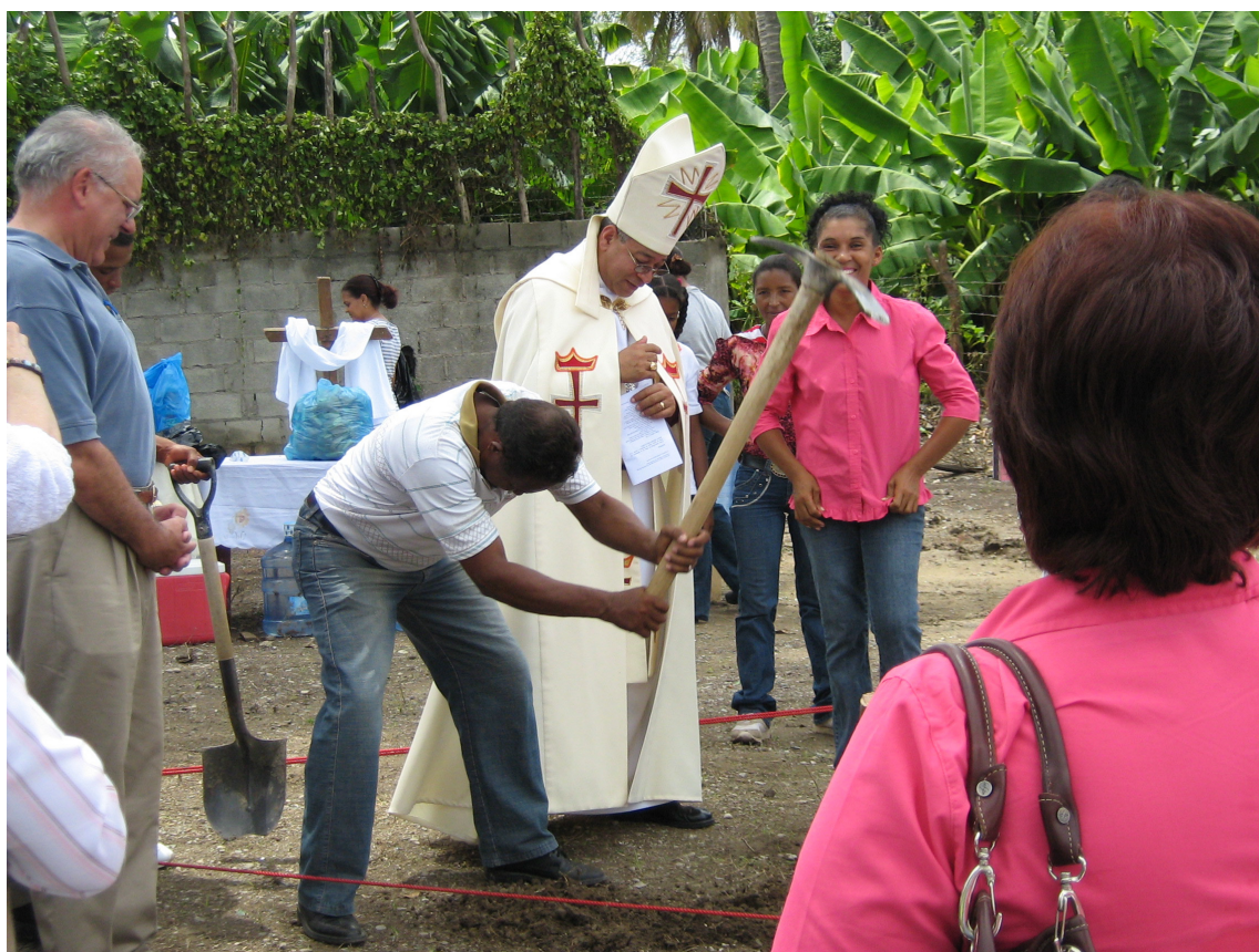
A Mission Team from St. Matthew's, Alliance, participated in a groundbreaking for a new Episcopal church in the Dominican Republic.
