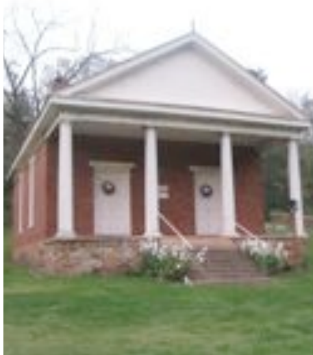
St. Luke's Episcopal Church, Pedlar Mills
