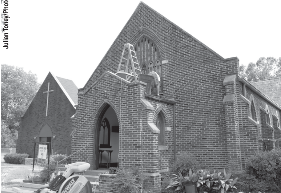
St. Thomas, Belzoni is getting a face lift. Many of the stained glass windows were in poor condition and were recently removed to be refurbished. Installation of the new windows began in late July.
