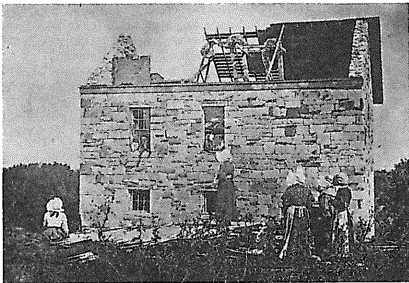
Damaged by Wind
