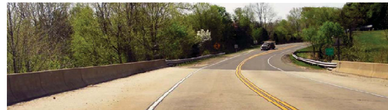
Typical bridge per VDOT's modern design standards.
