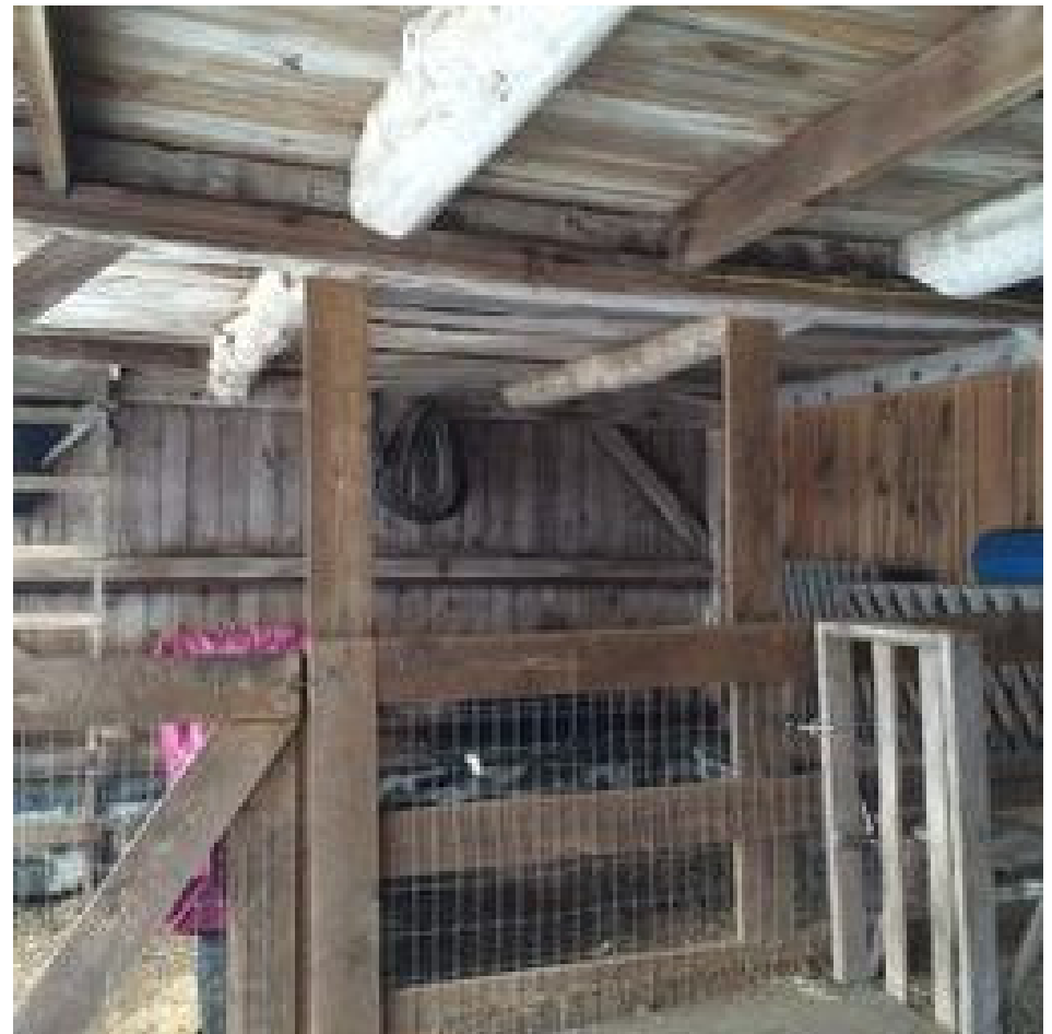
Interior views of North Barn bays
