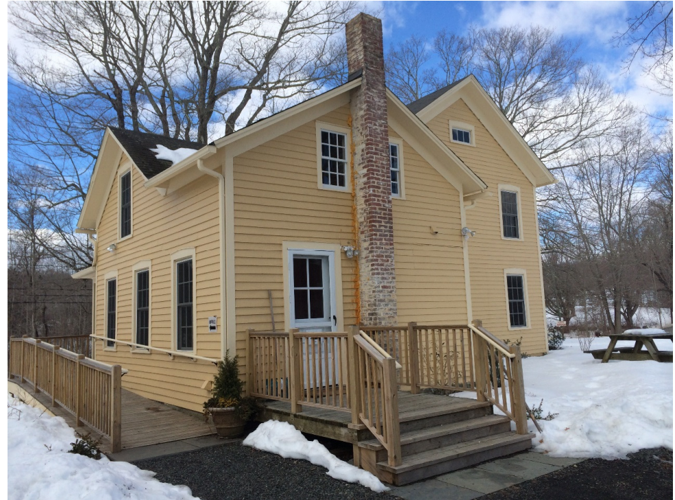
Rear of South Farm House
