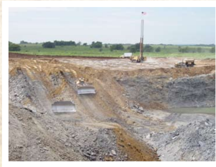
Bulldozers were used to move rock above coal at the Kelley Mine in Craig County, northeastern Oklahoma. The mine is mine number 8 in Figure 2 on page 11.
