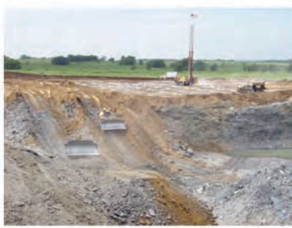
Bulldozers were used to move rock above coal at the Kelley Mine in Craig County, northeastern Oklahoma. The mine is mine number 8 in Figure 2 on page 11.
